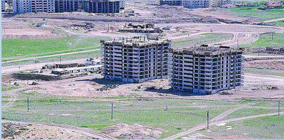
Multi-storey building construction (ten storey)
